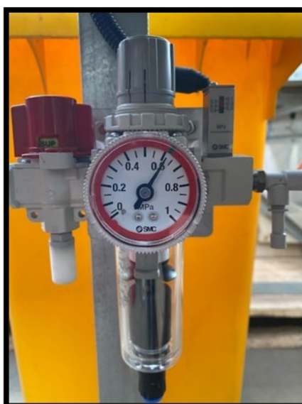
Figure 43. ART Air Pressure Gauge
