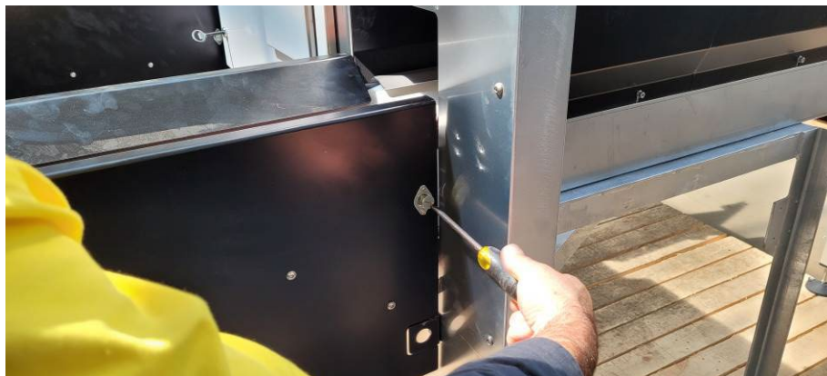
Figure 42. Safety Latches
