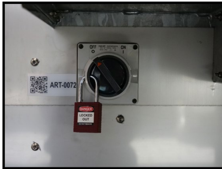
Figure 52. Power Isolator
